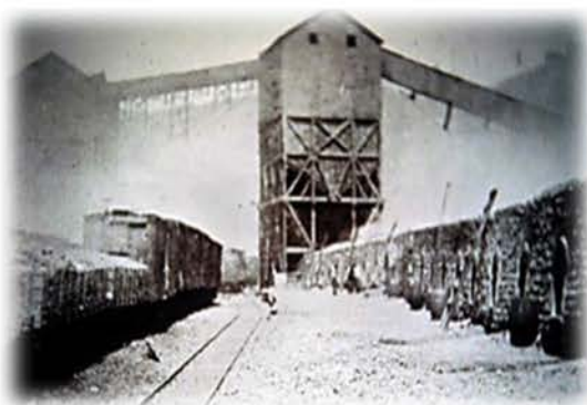
COKE OVENS AND A LOADING TIPPLE IN COKETON, WEST VIRGINIA IN THE 1890S.
